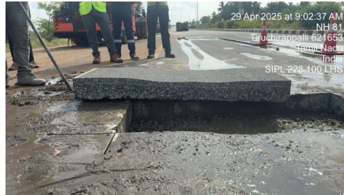
Rutting developed only on top bituminous layers
