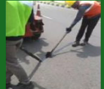
Crack seal with hot bitumen sealant
