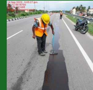
Crack seal with emulsion
