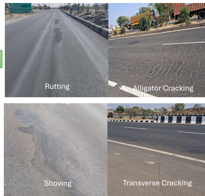
Typical Structural Failures
