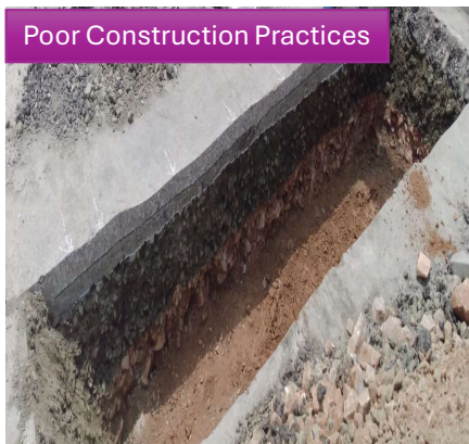
Poor Quality Soil for Subgrade
