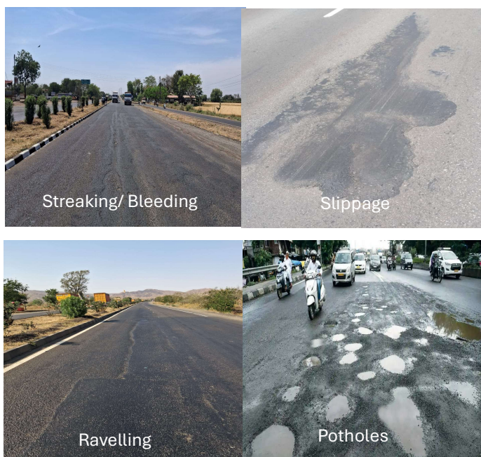
Typical Functional Failures
